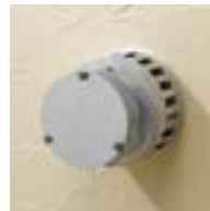
Balanced Flue (No chimney required) BF
