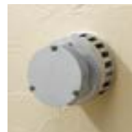
Balanced Flue (No chimney required)
